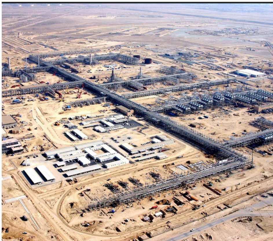
The Qatif Central Producing Plants in Saudi Arabia. Photo courtesy of Saudi Aramco.
