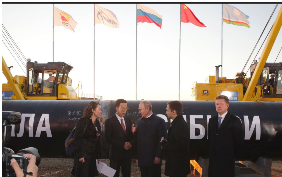
Russian President Vladimir Putin and Chinese Vice Premier Zhang Gaoli at the Power of Siberia pipeline construction launch on September 1, 2014. Source: Gazprom / RIA Novosti / Alexey Nikolsky
