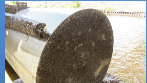
Valley Power Plant, Milwaukee, WI
