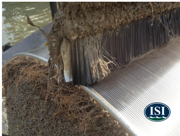
Figure 3. Intake Screens, Inc. Mechanical Brush-cleaned Screen Operating in Estuarine Hudson River
