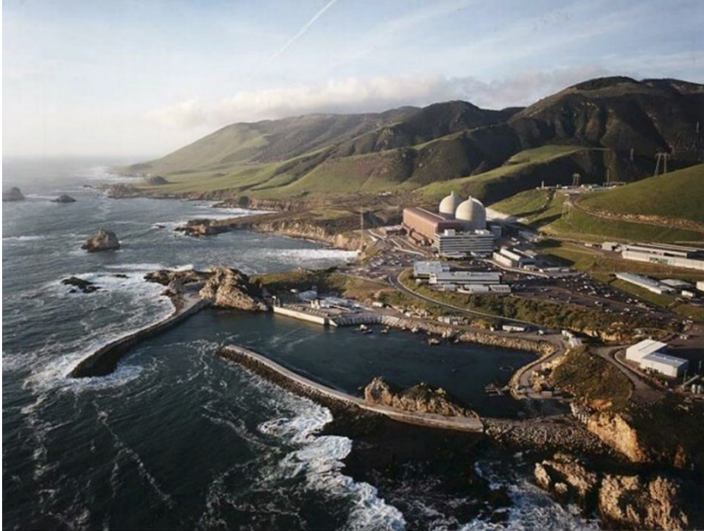
Figure 13. Aerial view of DCNPP, with Crowbar Canyon in the background.
